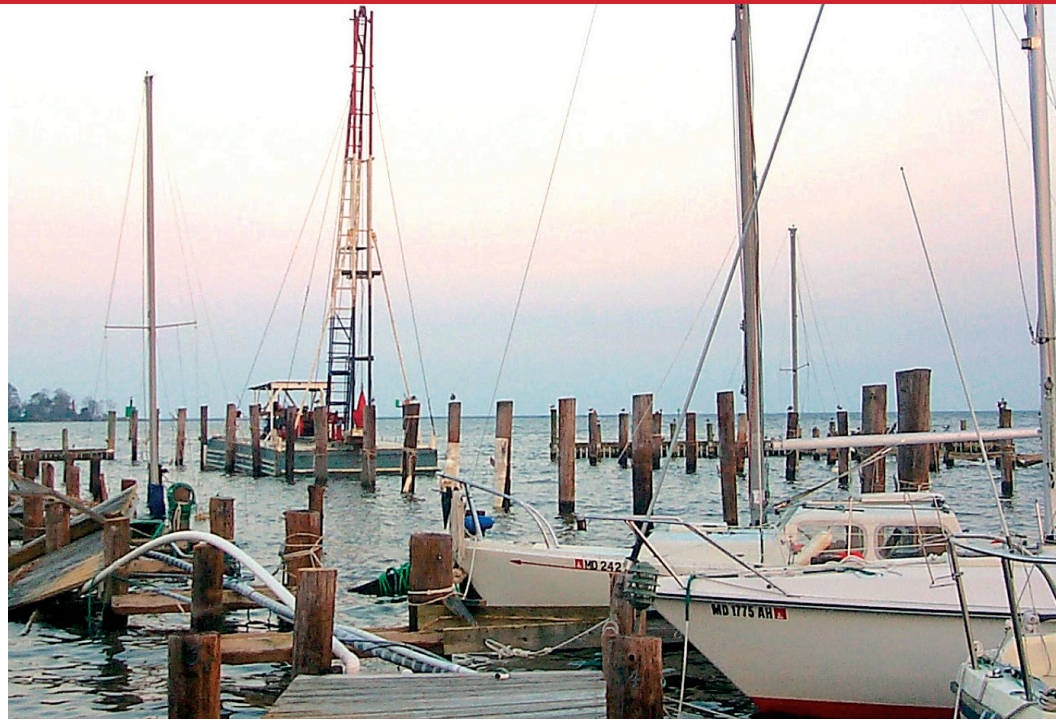
A storm surge during Hurricane Isabel combined with normal high tides to overcome this low-lying breakwater. The protected harbor then became an open bay and many of the boats in the harbor either sank or were badly damaged.
